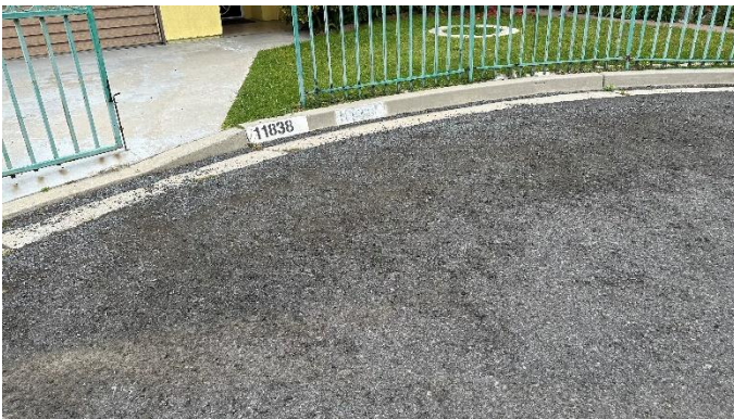
Picture 1: Raveling in front of 11838 Hermosura Street
